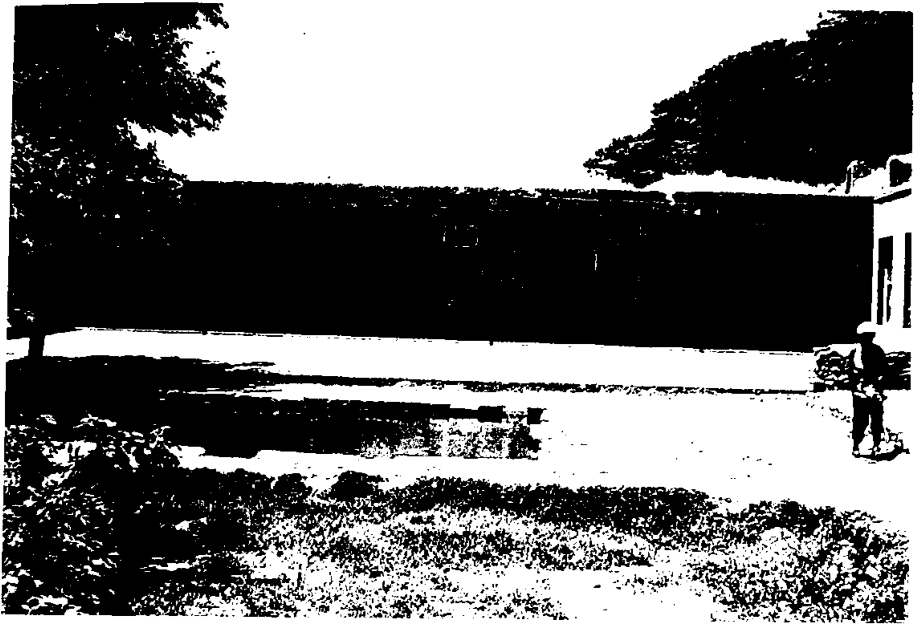
The somewhat dilapidated courtyard of the khānaqāh of Karukh. The pond is said to contain holy fish (B. Utas, 1978).
