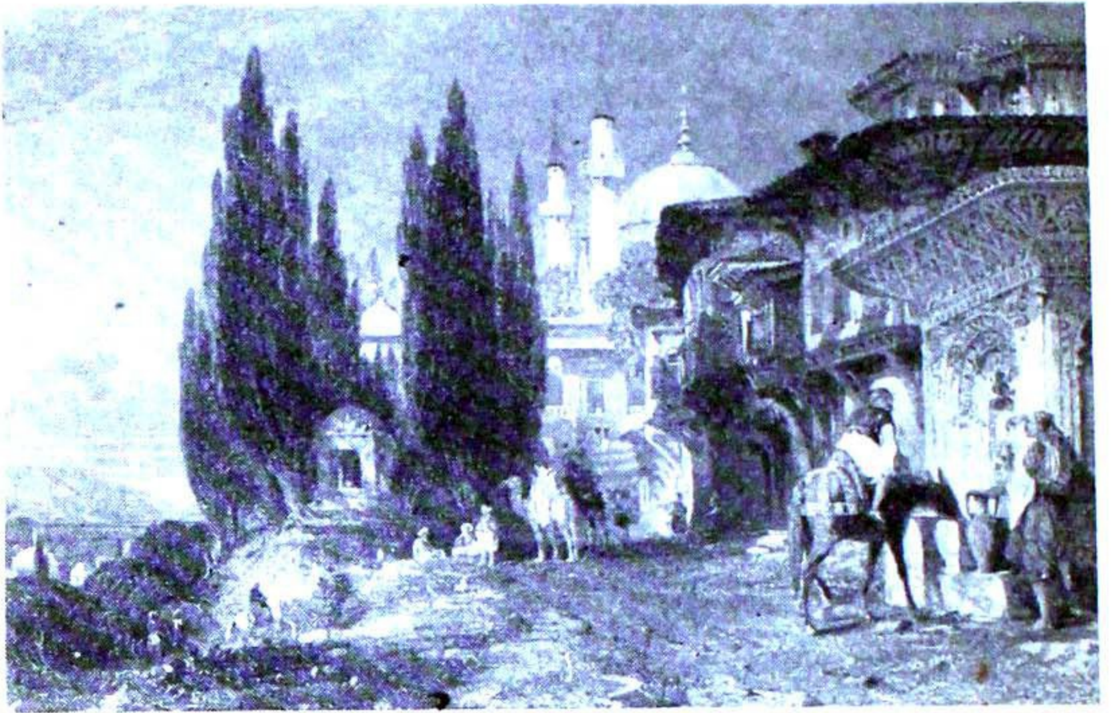
Buildings at Brusa.
