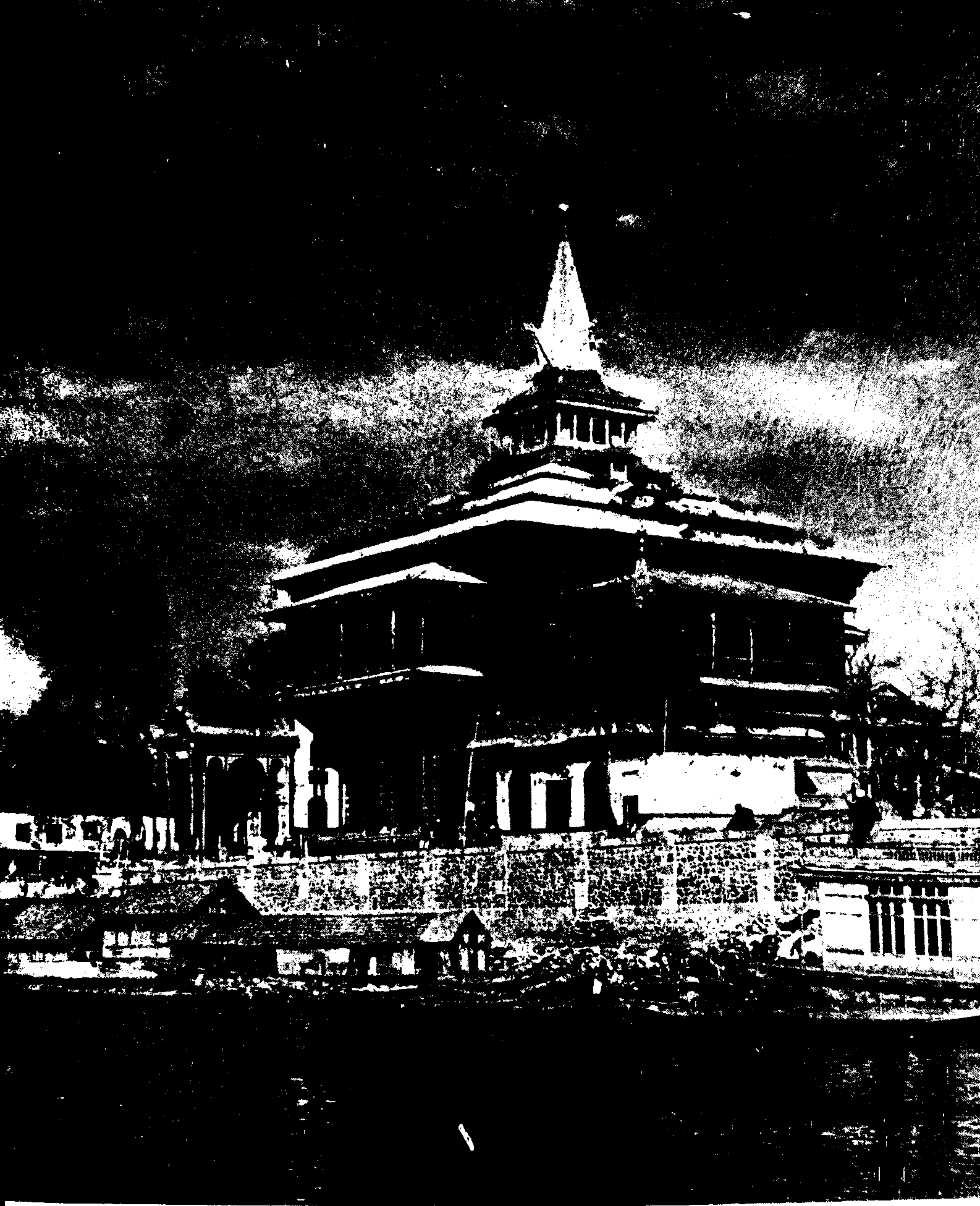
Shah-i-Hamadan Mosque in Srinagar (Kashmir) is another beautiful specimen of the distinctive architectural style of Kashmir mosques in wood.
