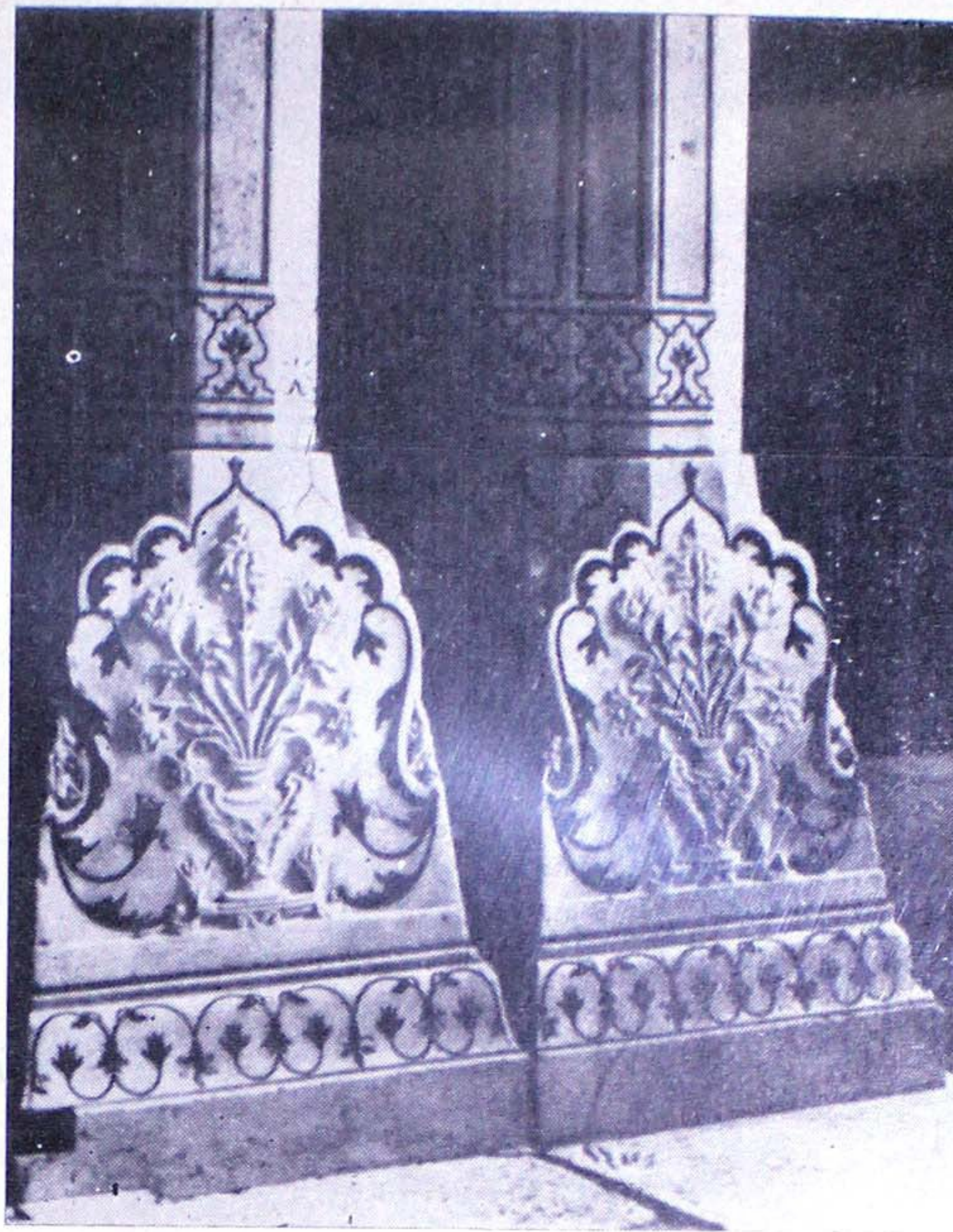
Floral design in bas relief & inlay work on marble column bases, Diwan-i-Khas, Agra Fort
