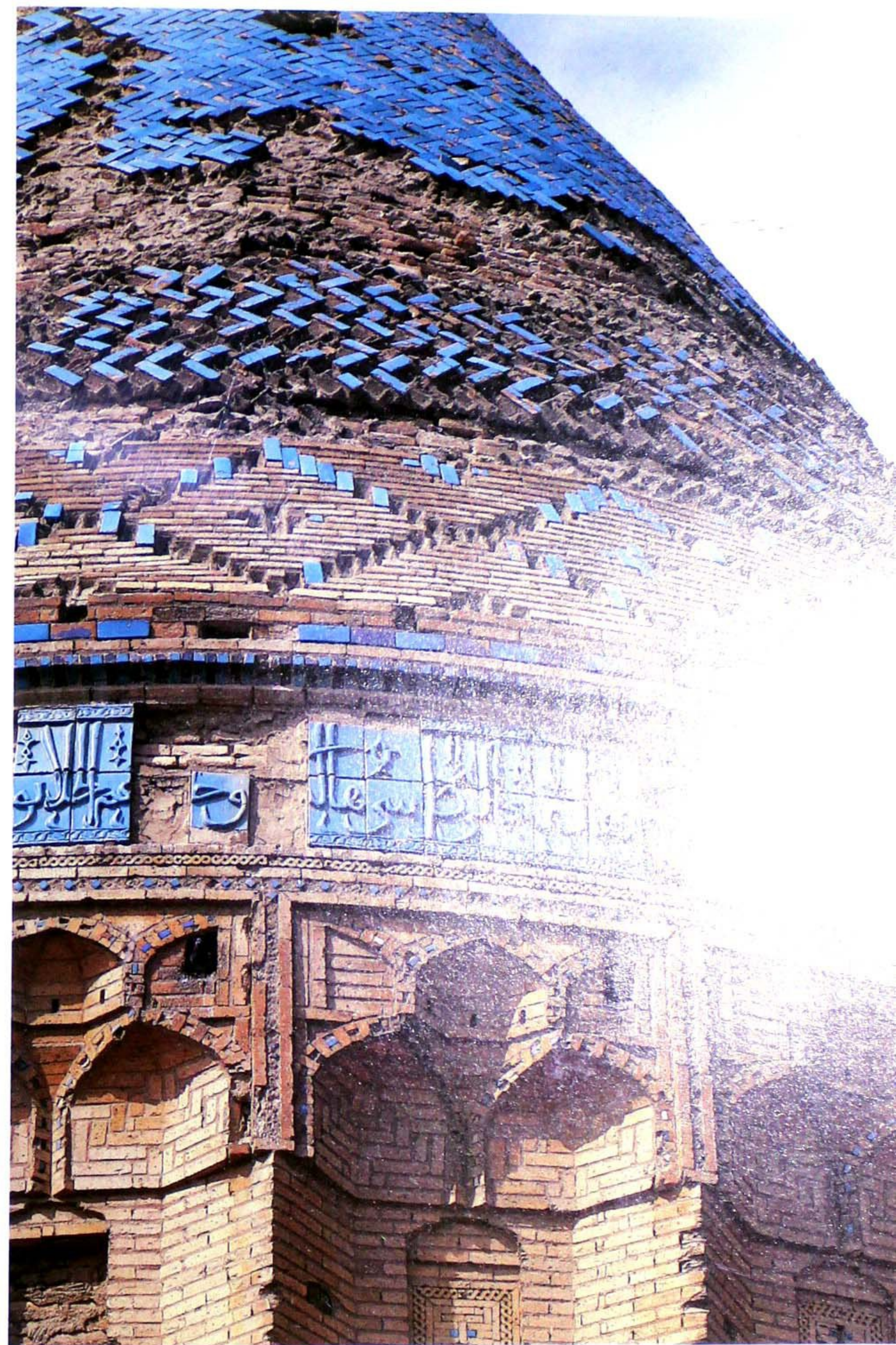
Detail of the Tekesh mausoleum in Kunya Urgench, famed for its ornate brickwork and glazed terra-cotta inscriptions.
