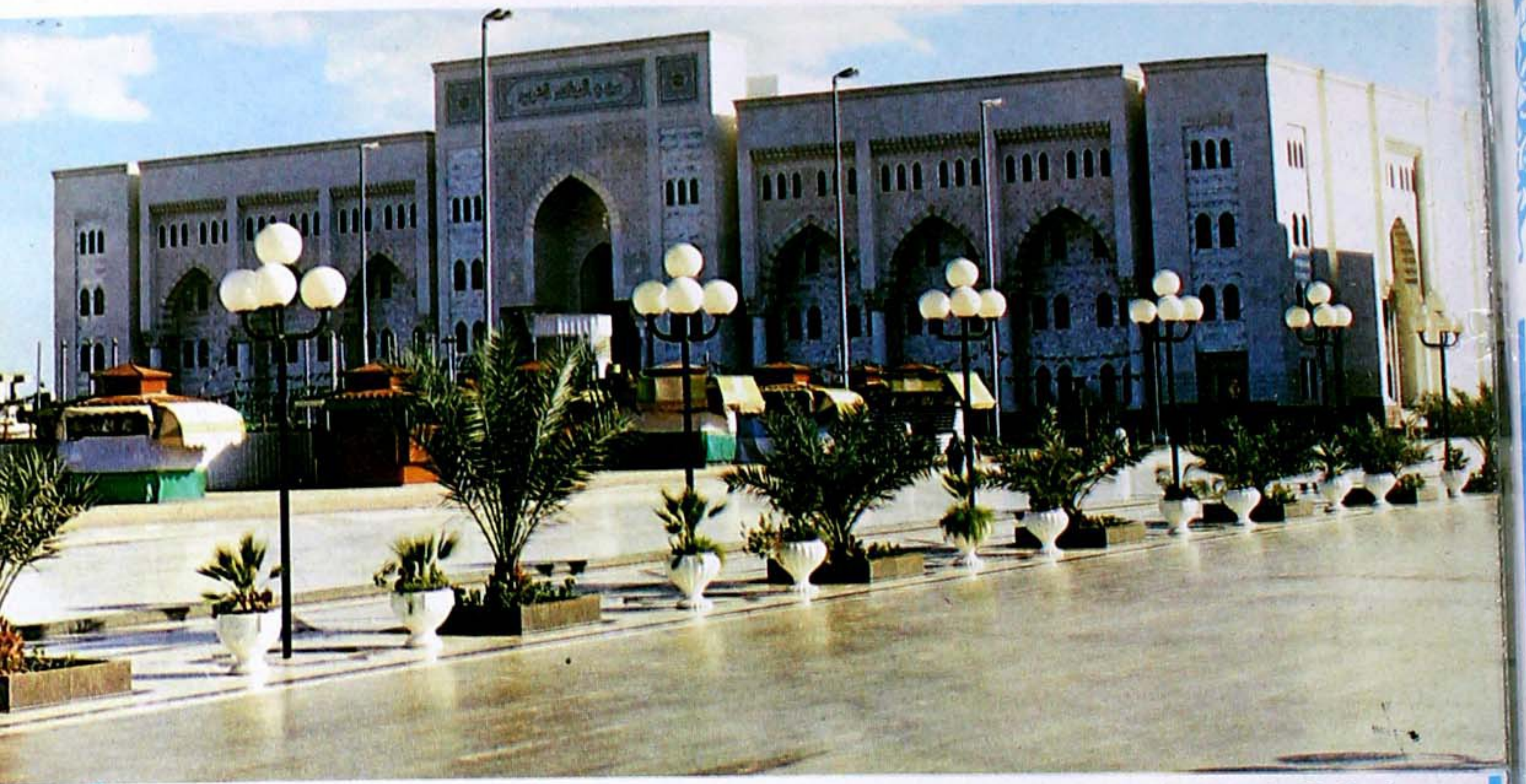
New Sharia Courts Complex in Madinah.
