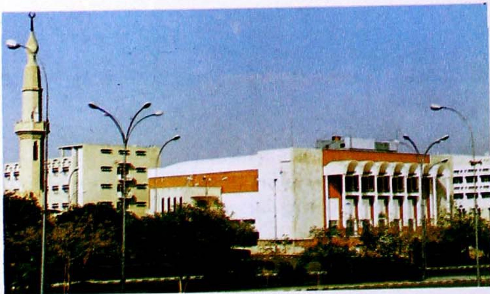
The Islamic University's Central Library Building
