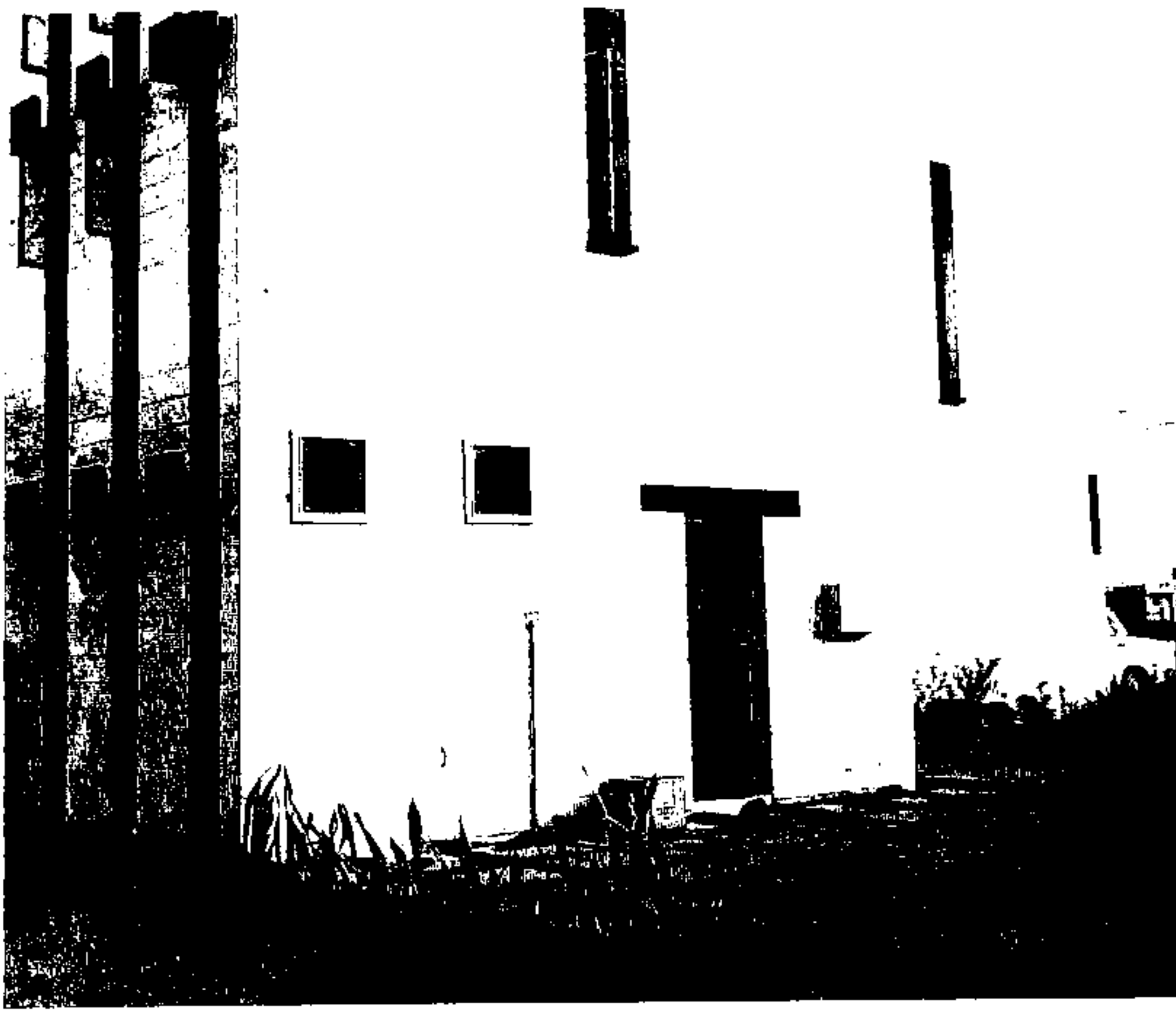
8.28 Commodore Haq's House, Karachi by Yasmeen Lari. The stark simplicity is the result of a painstaking refinement of plan and structure, clearly expressing the discipline of load bearing block work and spanning concrete.
