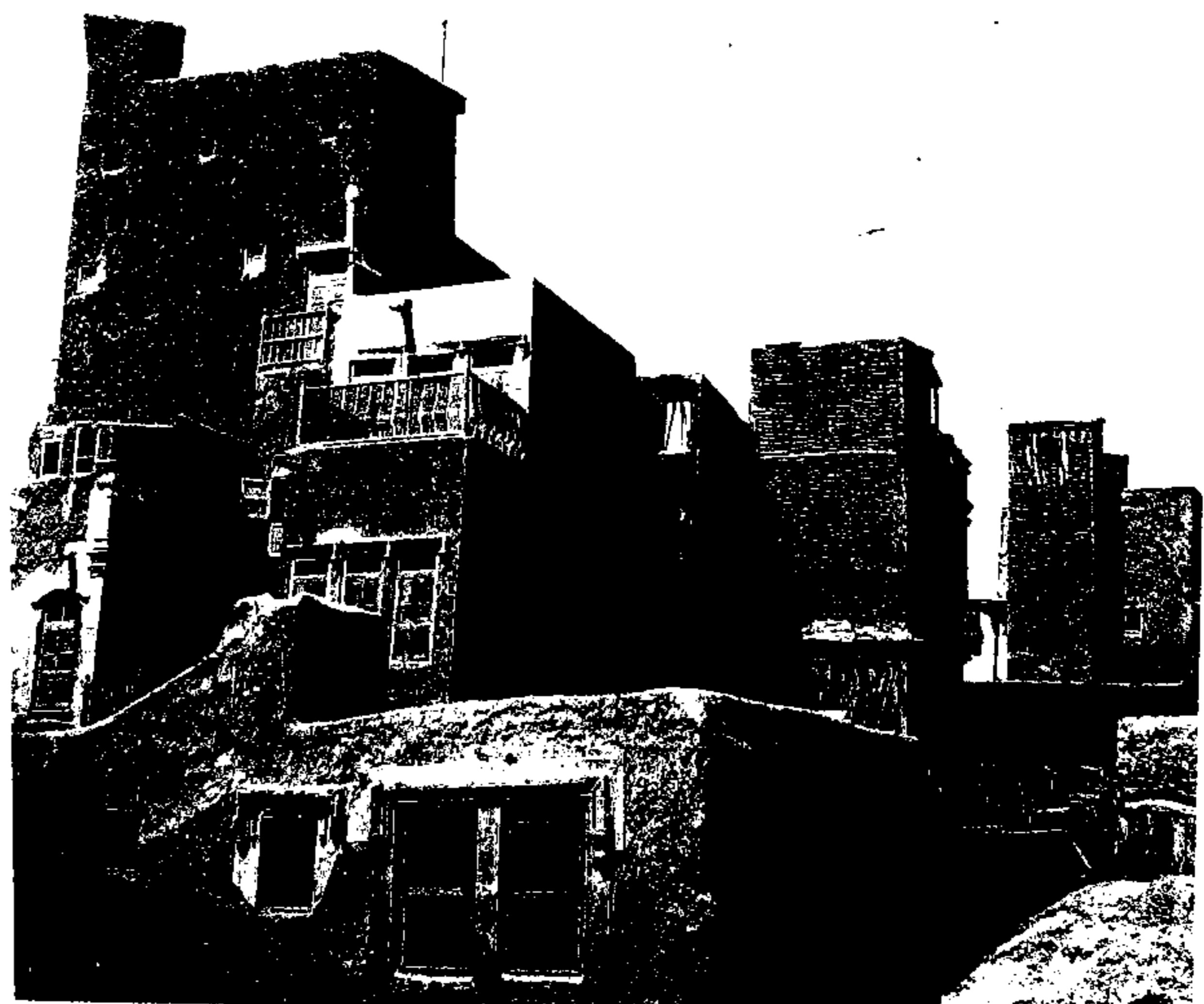
7.1, 7.2 and 7.3 Townhouses and wind-catchers, Thatta. Thatta presents a rare combination of urban verticality with rustic wattle and daub surfaces. On every roof is perched a wind-catching device, known locally as a "mungh".
