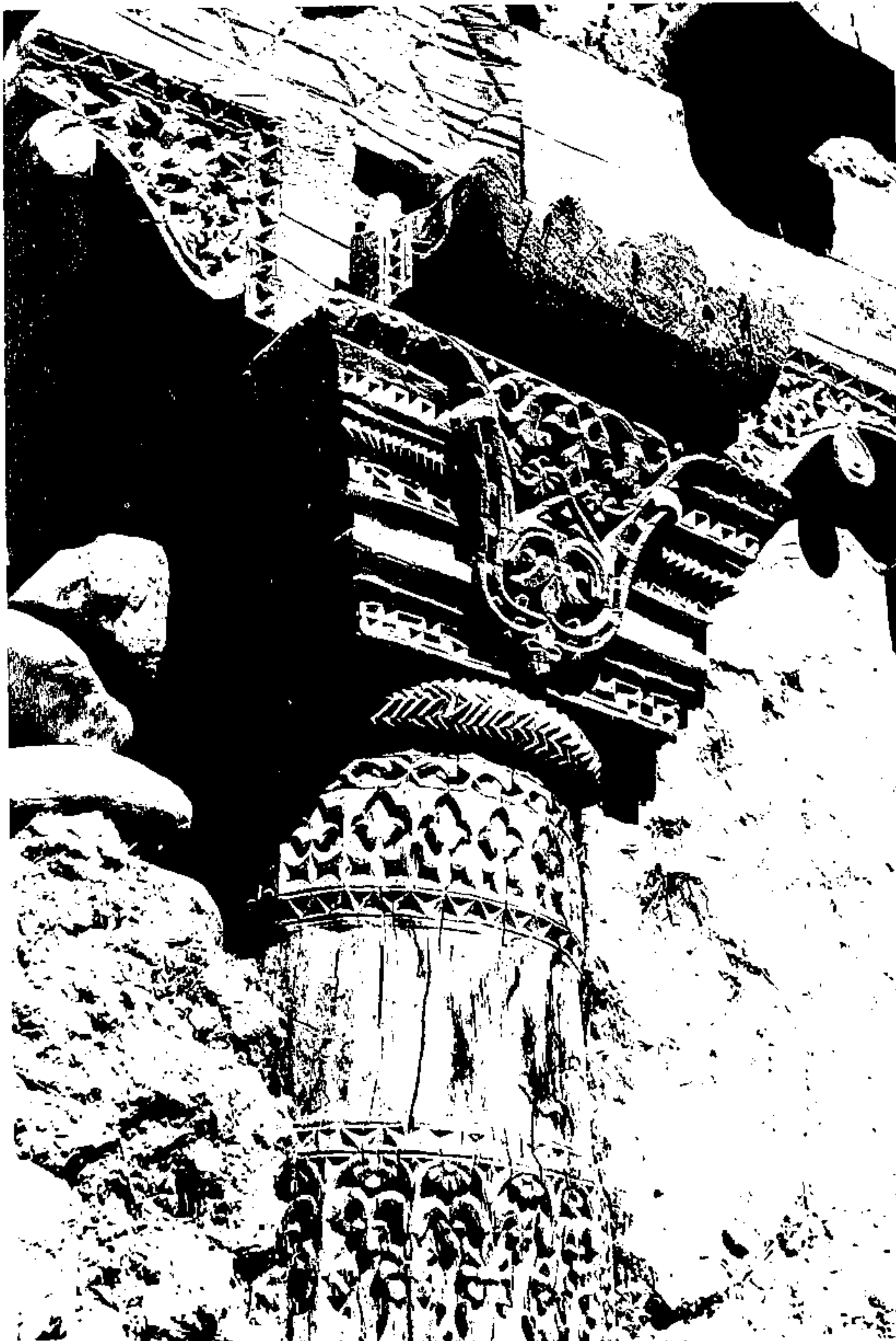
7.38 Timber Column, Skardu. If the rustic brutalism of the structure of this shrine in the remote valley of Shigar appear crude, it is due only to its impoverished state of preservation rather than to a lack of sympathy or respect for the material.
