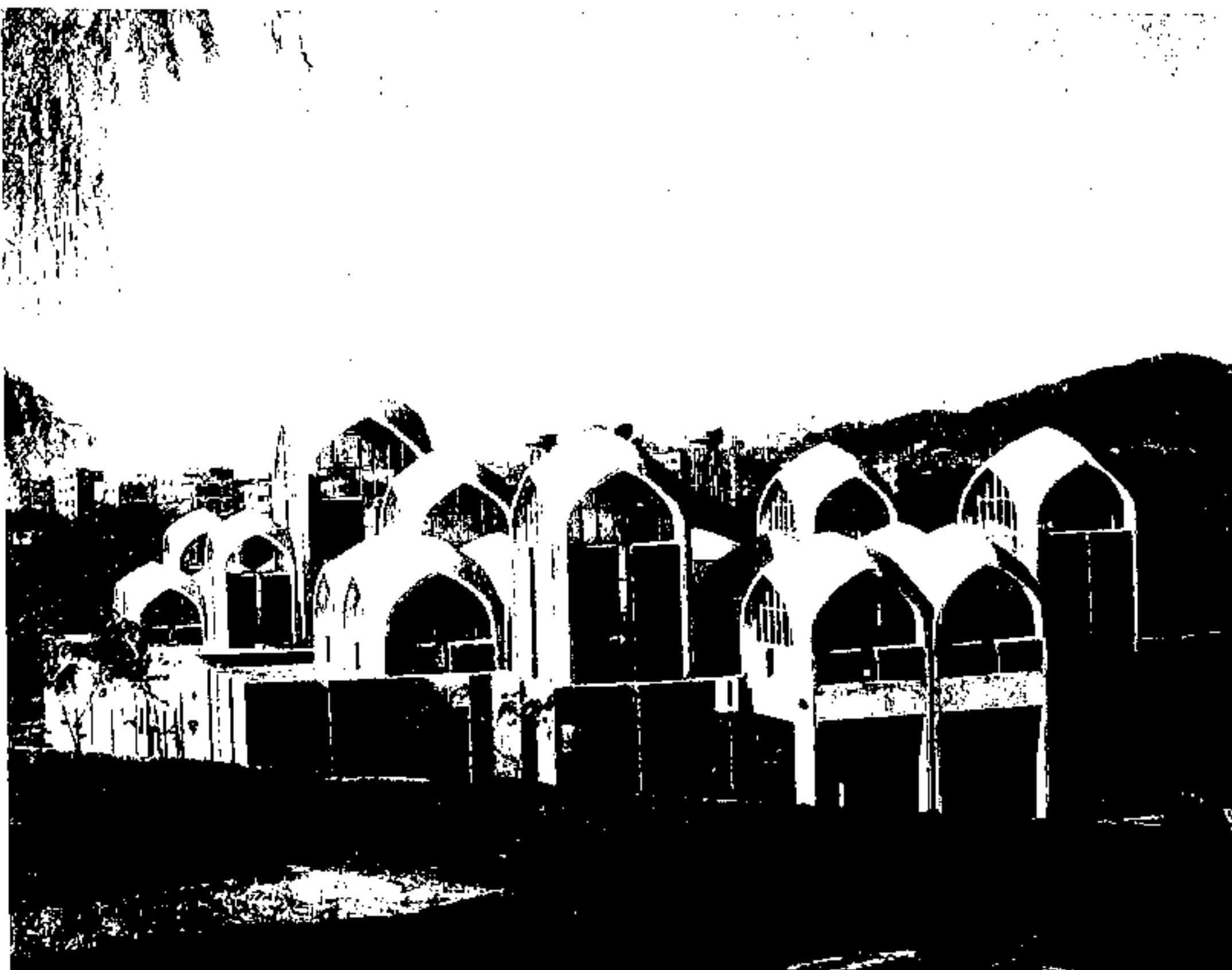
8.40 Neighbourhood Mosque, Islamabad. Anwar Saeed, a prolific designer of community and public authority buildings, is a disciple of the constructivist, purist or elementarist school within the Modern Movement.
