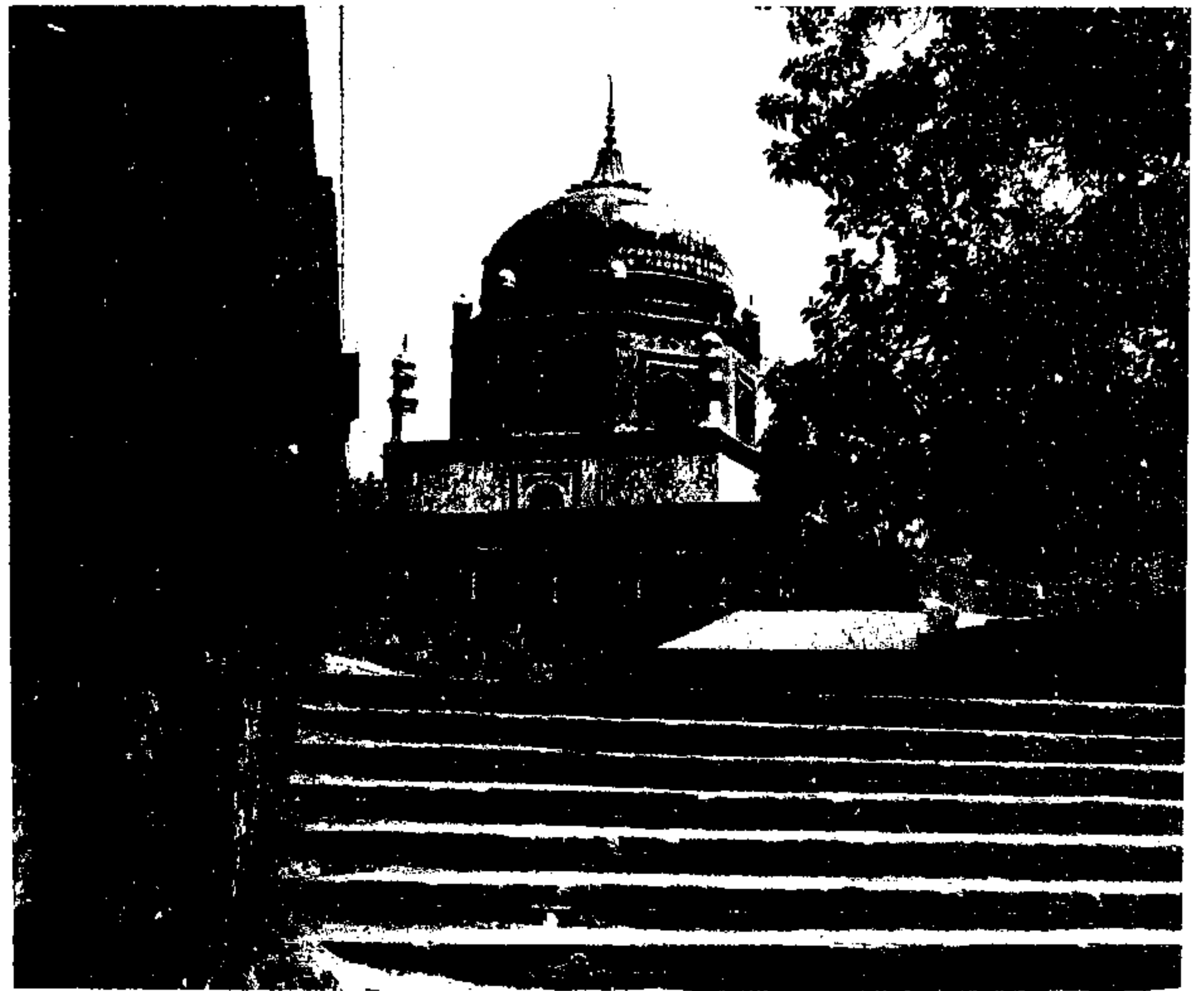
3.8 and 3.9 The essential form of the Tombs of Shah Baha ul-Din Zakariya and Shah Shams Sabzwari with their square plans, octagonal drums, a central dome and corner minarets, establishes a type of mausoleum building which was to endure for 700 years.
