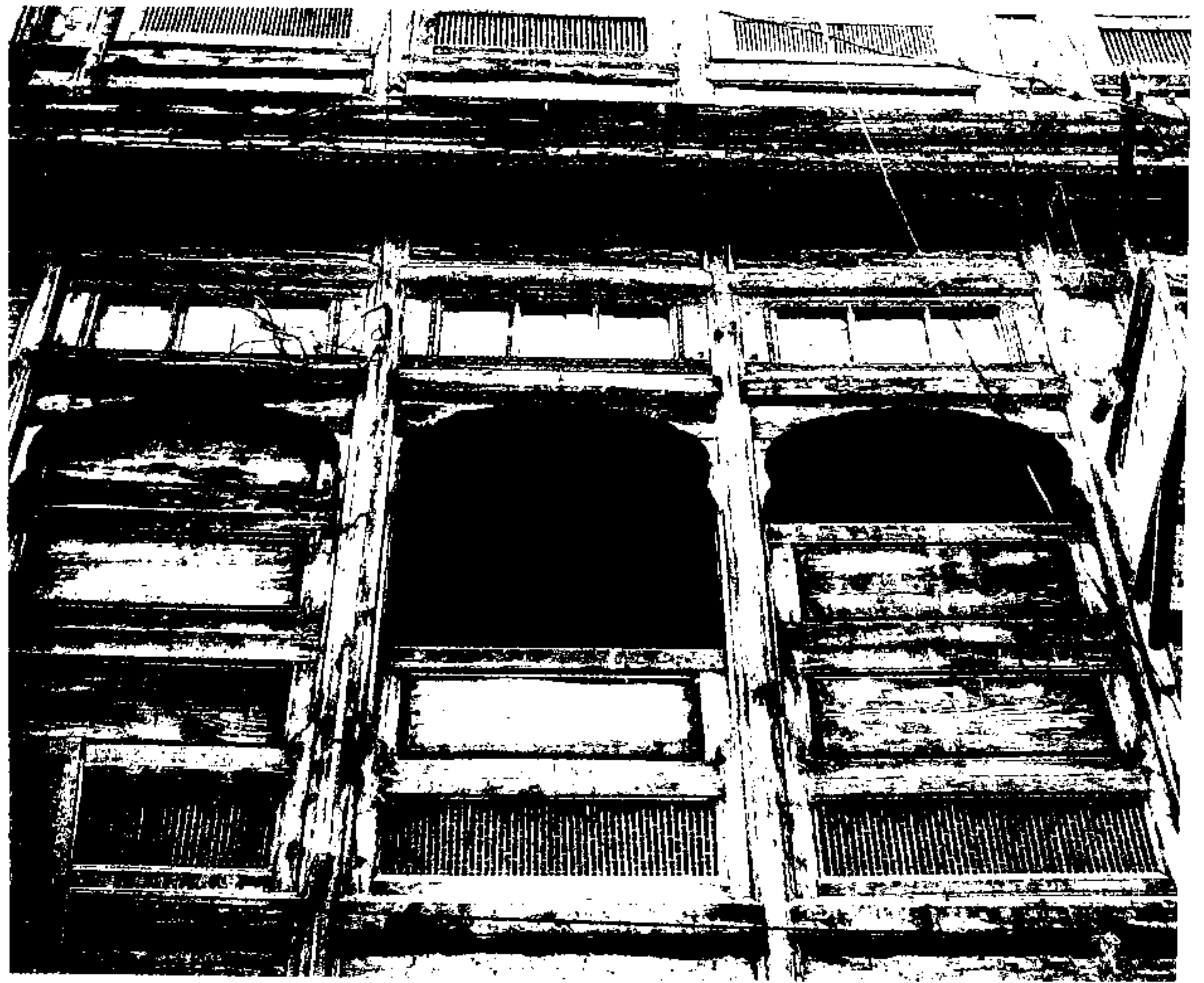
7.35 and 7.36 Balconies, Sarafa Bazar, Peshawar. In Peshawar it is not unusual to find continuous multi-storey street facades of pure timber curtain walling with vertically sliding shutters.
