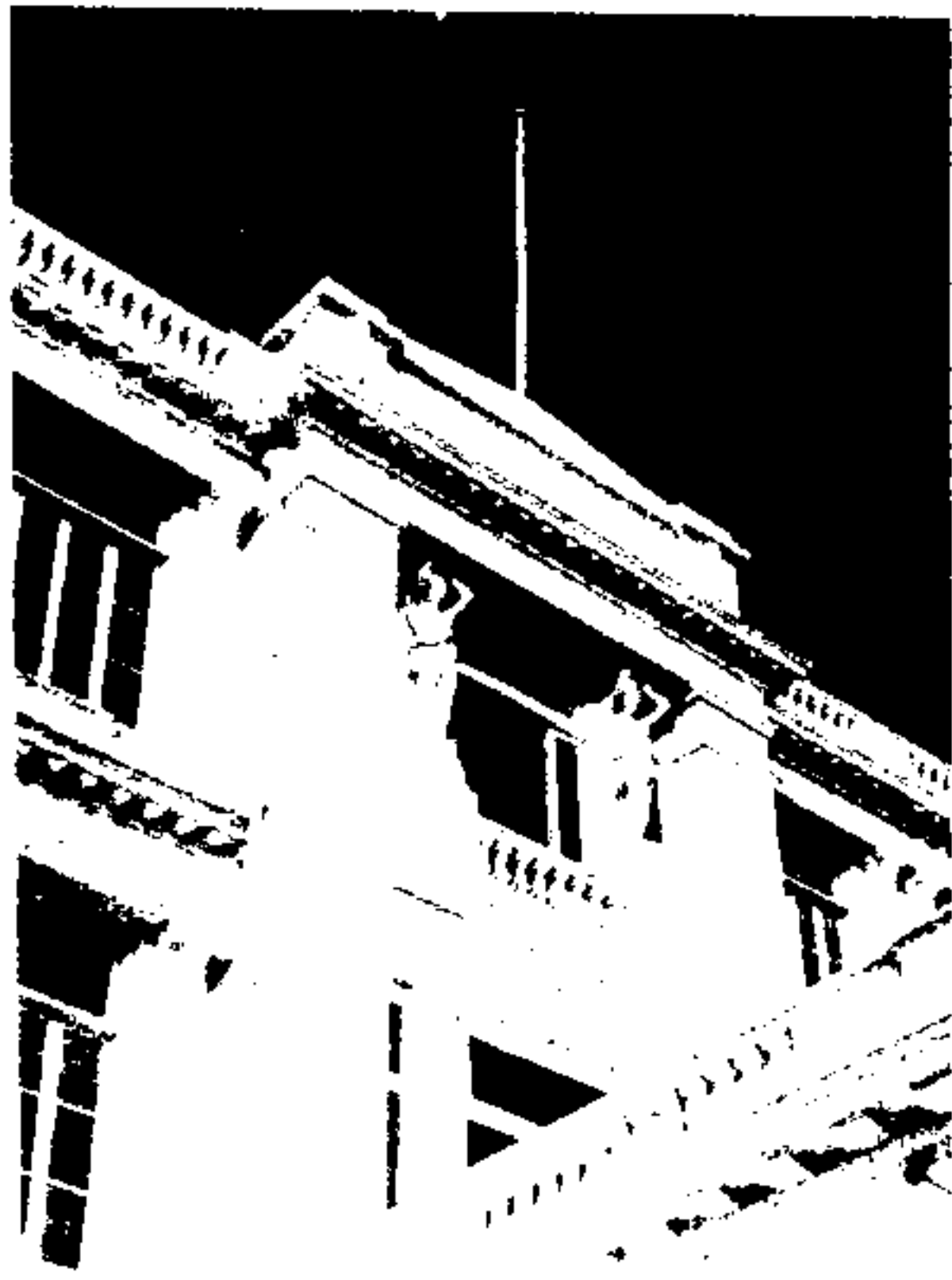
6.6, 6.7 and 6.8 The reverberations from the battle of the styles were felt throughout the colonial territories and left behind a litter which included everything from Gothic steeples (6.6 Frere Hall) to classic revival (6.8 Sind High Court) and Palladian villas (6.7 Palace Hotel).
