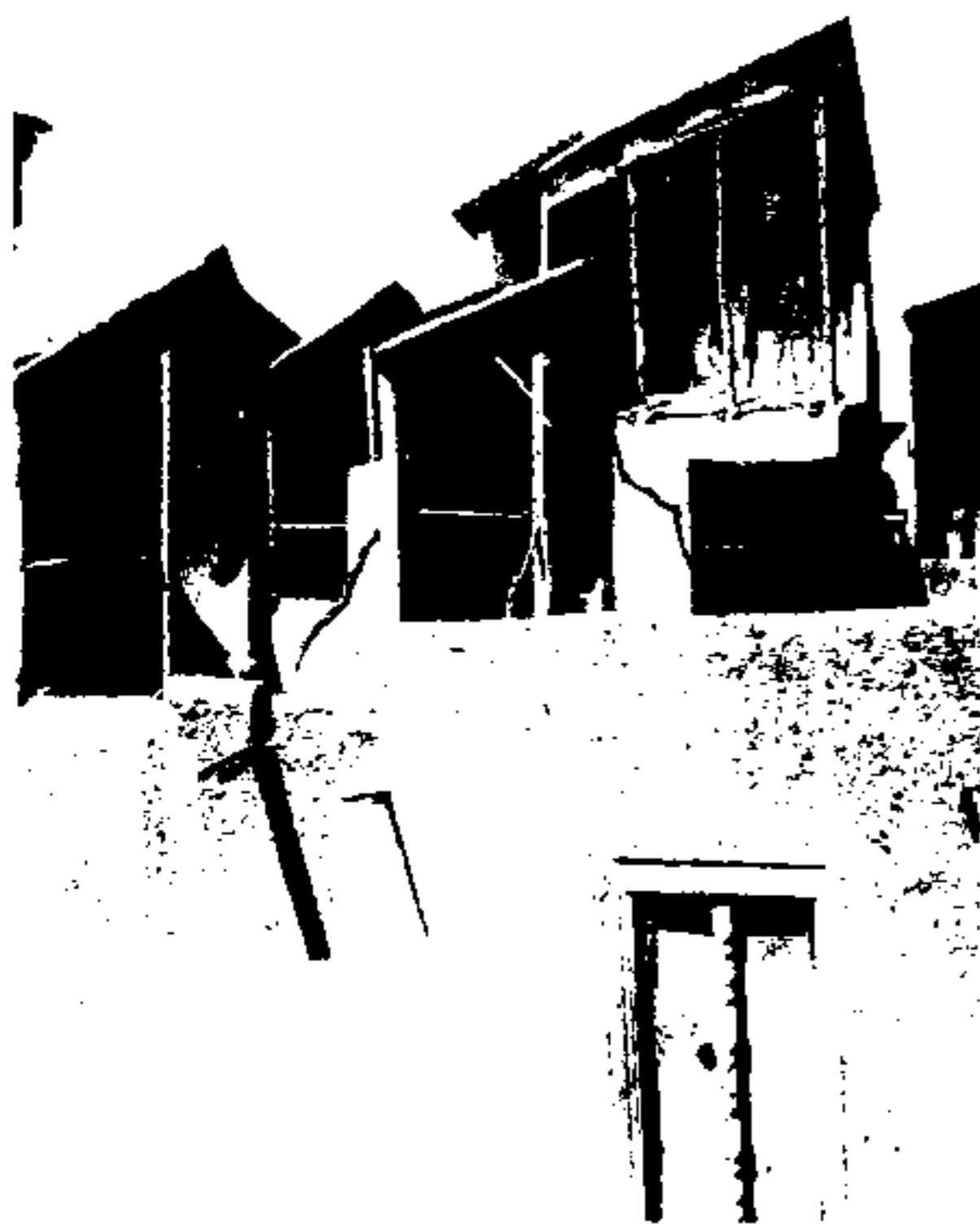
7.1, 7.2 and 7.3 Townhouses and wind-catchers, Thatta. Thatta presents a rare combination of urban verticality with rustic wattle and daub surfaces. On every roof is perched a wind-catching device, known locally as a "mungh".
