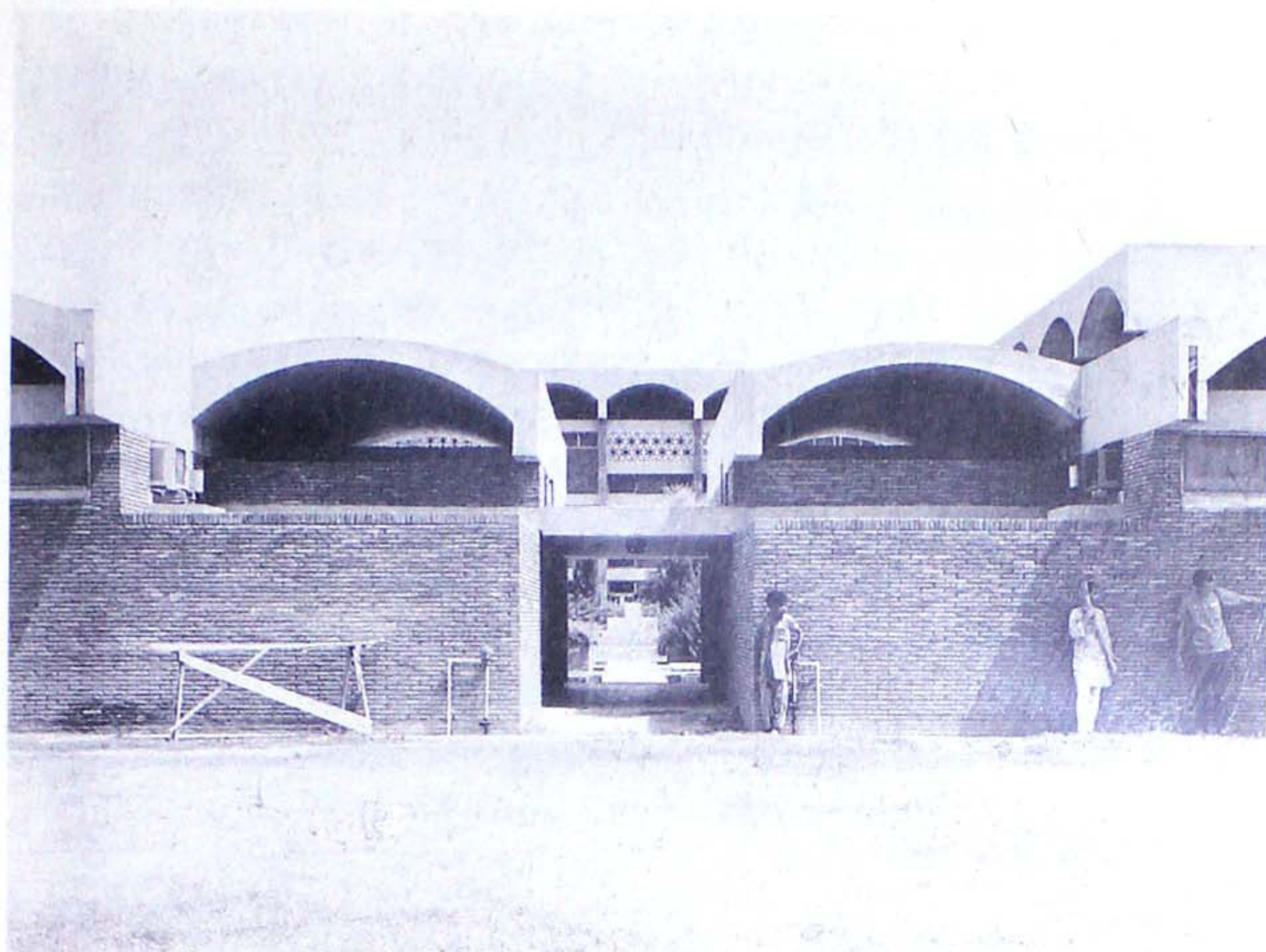
8.53 Government officers' Hostel, Islamabad, displays an intelligent application of traditional elements to contemporary building. It is probably the most satisfying individual building in Islamabad.
