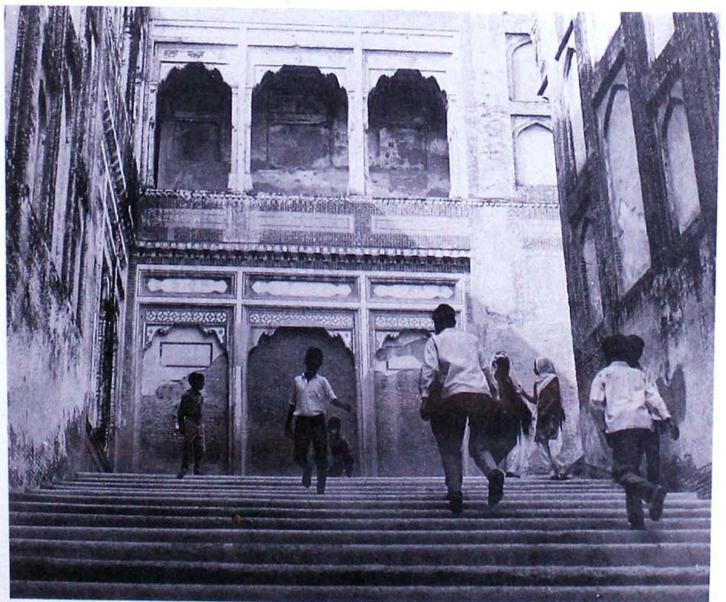
4.15 Hathi Pol, Lahore Fort. The royal passage from Hathi Pol gate to the outer court of Shish Mahal was built by Shah Jahan in 1632. It includes a flight of giant steps called Hathi Paer or Elephant Path.
