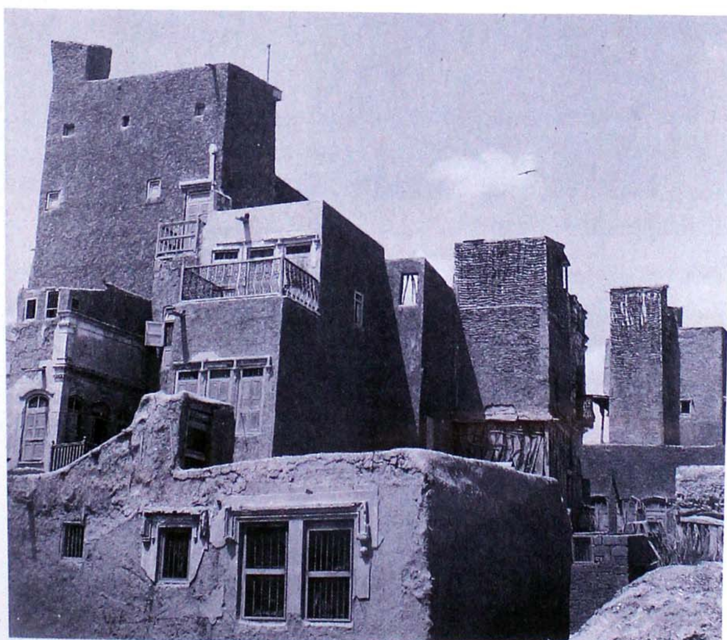
7.1, 7.2 and 7.3 Townhouses and wind-catchers, Thatta. Thatta presents a rare combination of urban verticality with rustic wattle and daub surfaces. On every roof is perched a wind-catching device, known locally as a "mungh".
