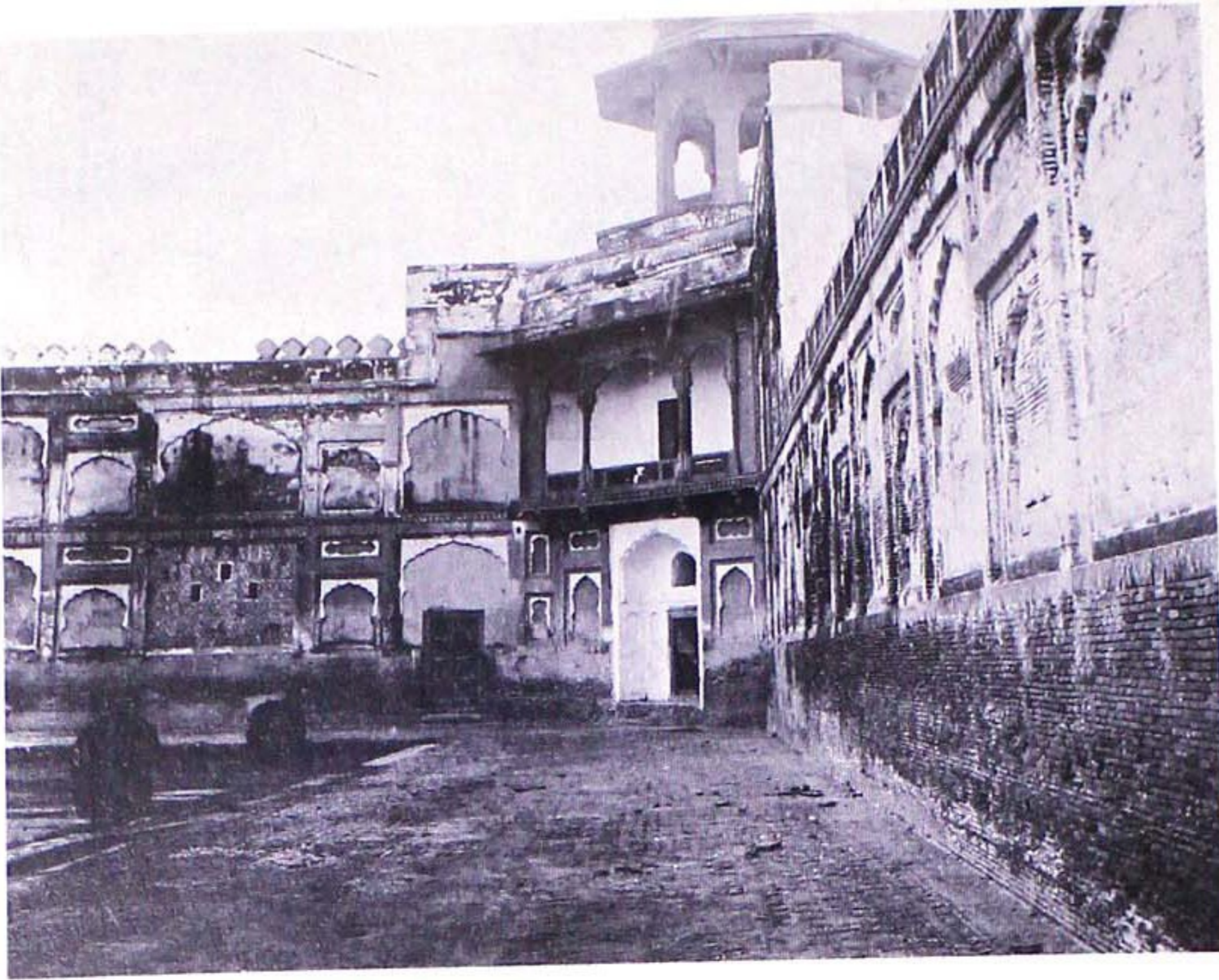
4.24 Corner of outer wall of Shalamar Bagh.
