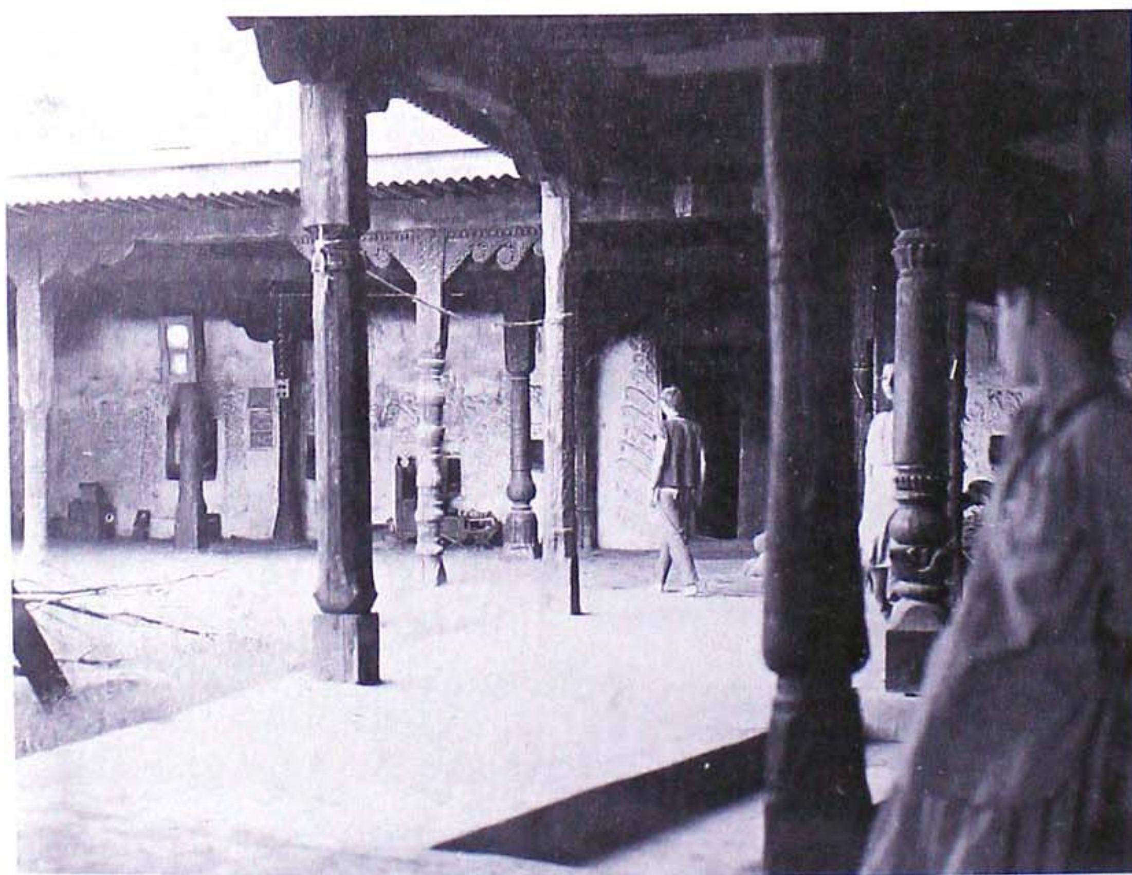
7.41 and 7.42 Mosque, Madyan. The central mosque at Madyan is a classic model of architectural discipline and refinement. Its carved scroll capitals emphasise elegance. Designs in relief on the mud-plastered west wall strikes a curious note of gaiety. The serenity of the courtyard enclosed by gracious loggias, testifies to the keen architectural sensibilities of its builders.
