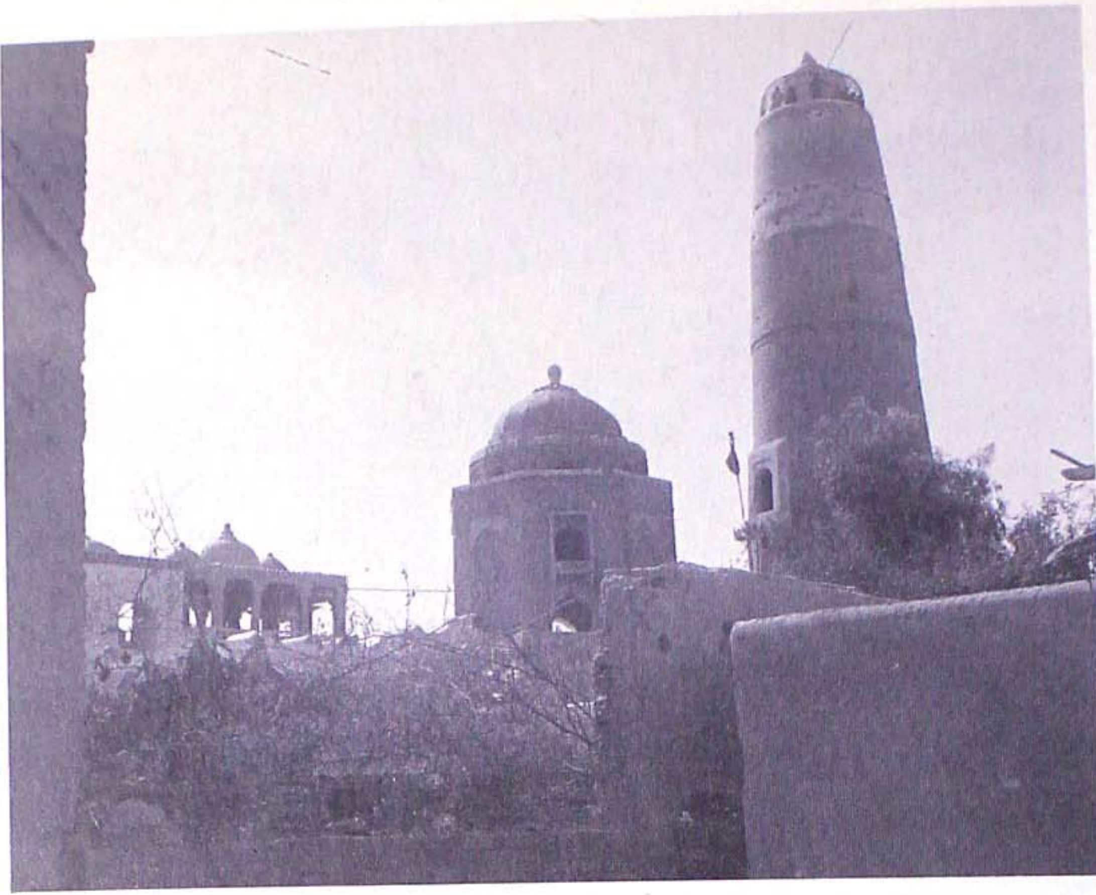
5.35 Tower and "Aram Gah" of Mir Ma'sum, Sukkur. Much of Mir Ma'sum's prolific building activity was devoted to public amenities such as bridges, rest-houses, inns, wells and river markers. The tower at Sukkur is intended for observing the countryside around. The domed octagonal 'Aram Gah' or rest-house is likewise a secular building.
