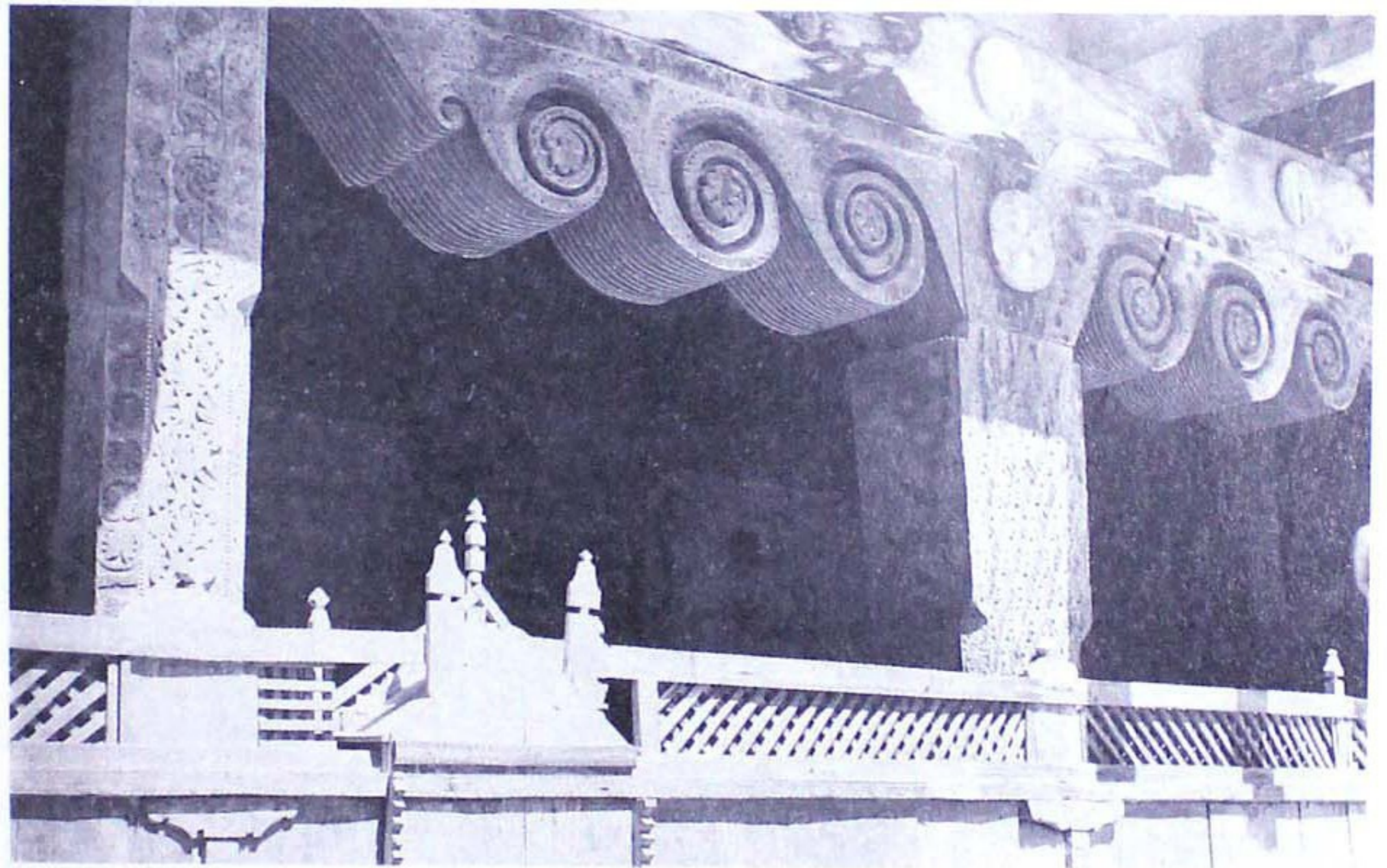
7.39 and 7.40 Mosque, Kalam and detail. Interlocking logs at the corners of a square tower are in fact an integral part of a highly developed craft tradition. Such powerful carving as gigantic scrolls of enormous capitals in the great mosque at Kalam, was probably performed as an act of worship for the glory of God.
