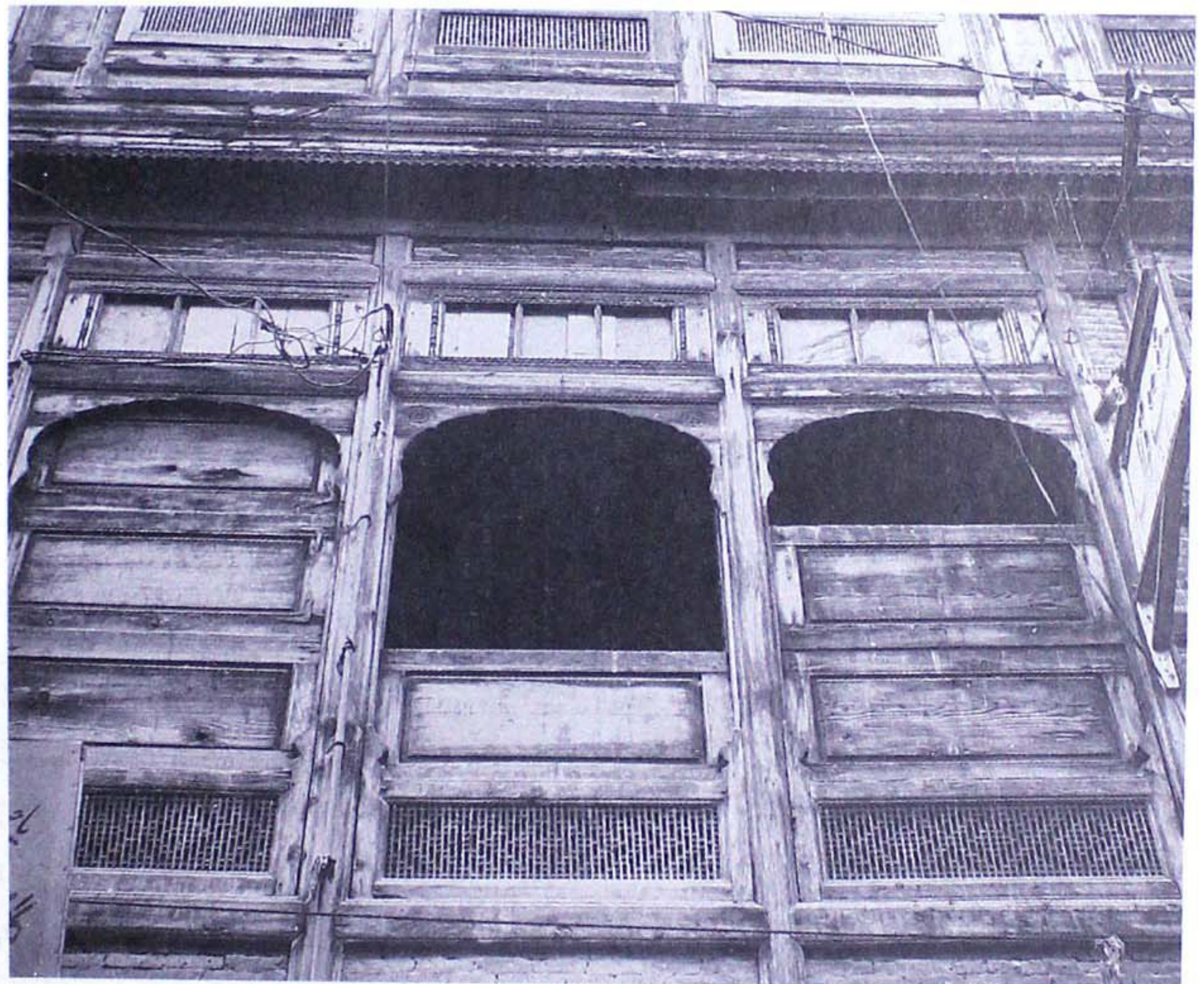
7.35 and 7.36 Balconies, Sarafa Bazar, Peshawar. In Peshawar it is not unusual to find continuous multi-storey street facades of pure timber curtain walling with vertically sliding shutters.
